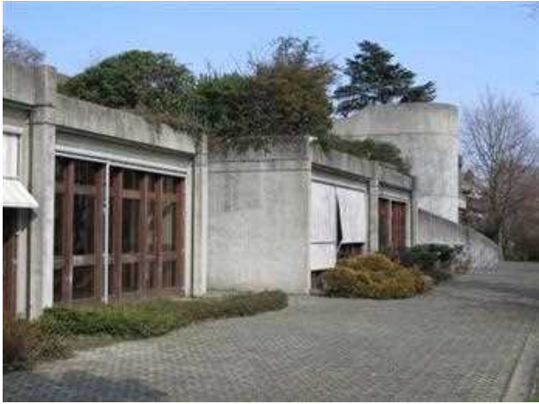
Fig. 108. Gymnase, façade sud.
